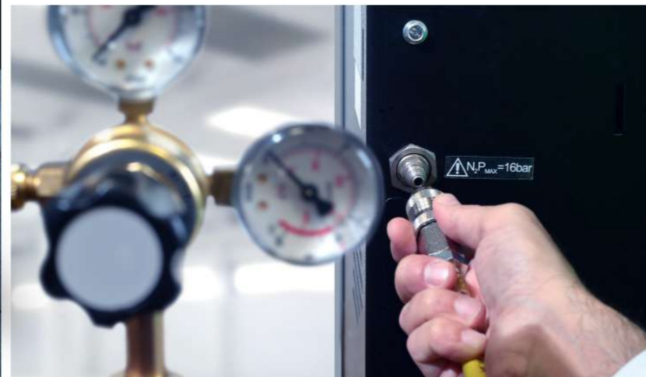
Nitrogen pressure control
